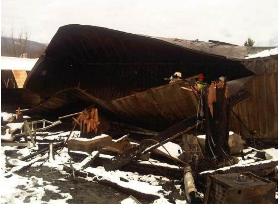
The photo below shows the folding of one the doors as it blew out of the latches and flew over 10m
